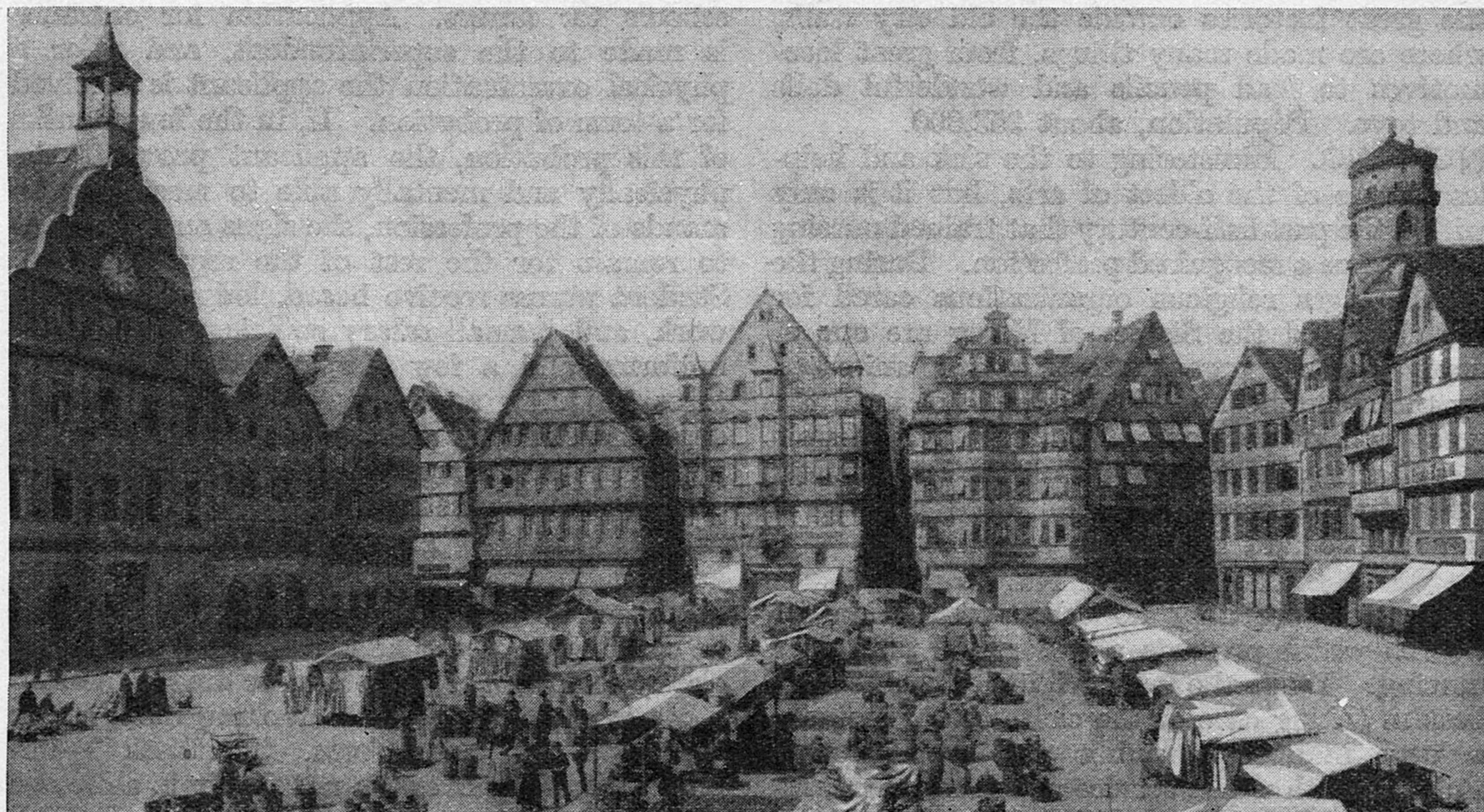
The Market-place in picturesque old Nuremberg, with the peaked gables of its tall and broad houses turned towards the street, carries us back to the Middle Ages. But not all these houses are old, for most of the citizens of Nuremberg, in building new houses, are careful to imitate the old ones, red-tiled roofs and all.
